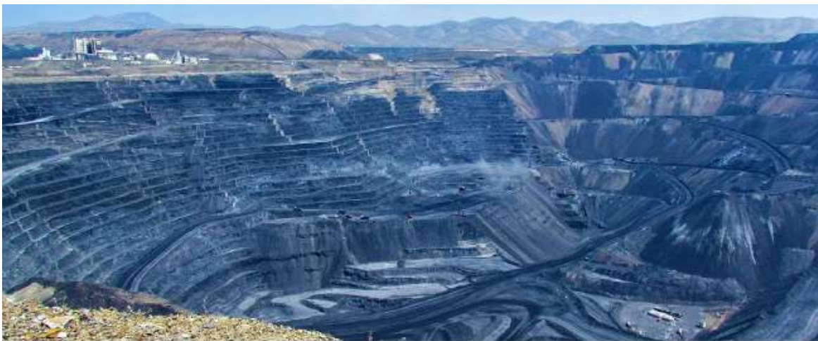
1.2: A gold mine on federal land in Nevada; example of commonly dug and facilitated mining worksites
