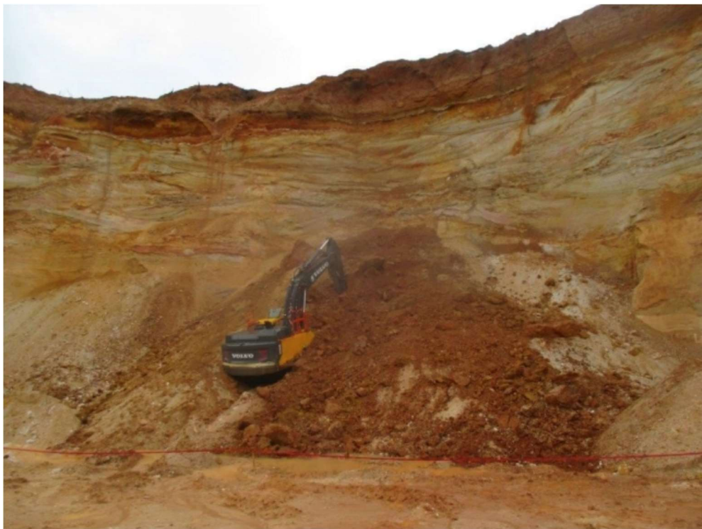
4.2: Failure to examine each angle of a highwall can lead to disaster; always take proper precautions
