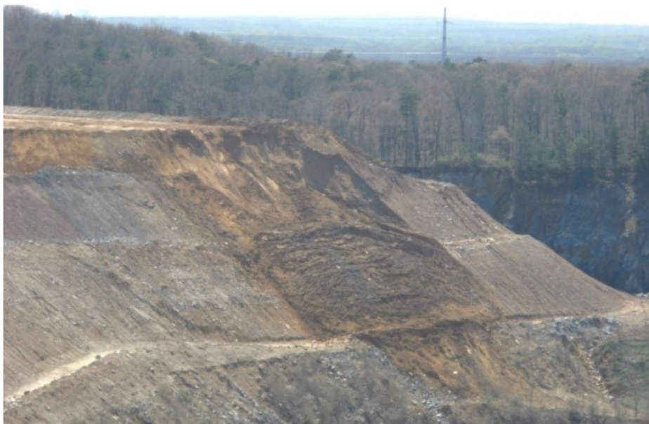
4.1: To avoid dangerous mining landslides (as seen above), use proper tools and methods when scaling any area of a mining worksite.
