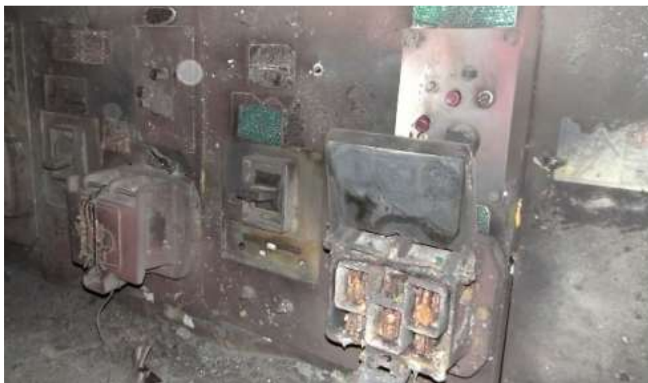
2.22: Aftermath of burnout breaker after arc flash accident
